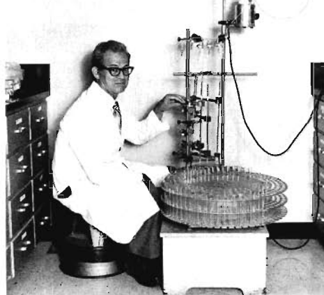
Using an ion exchange column and fraction collector to separate metabolites from human erythrocytes.
