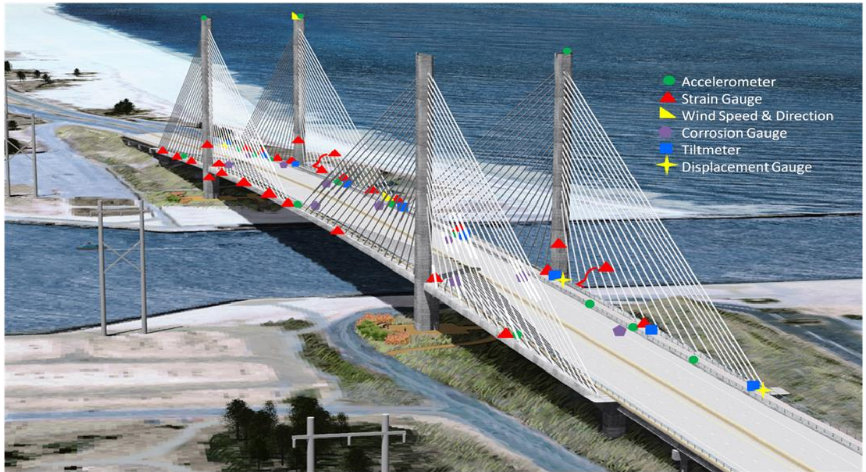
Indian River Inlet Bridge, Structural Health Monitoring System, Univ. Delaware (2012)
