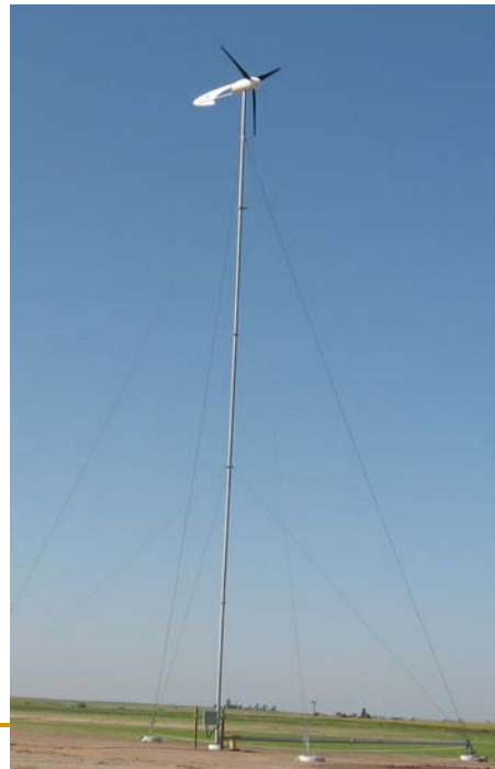
First turbine (4.2 kw) in Greensburg, at John Deere dealership model for community wind
