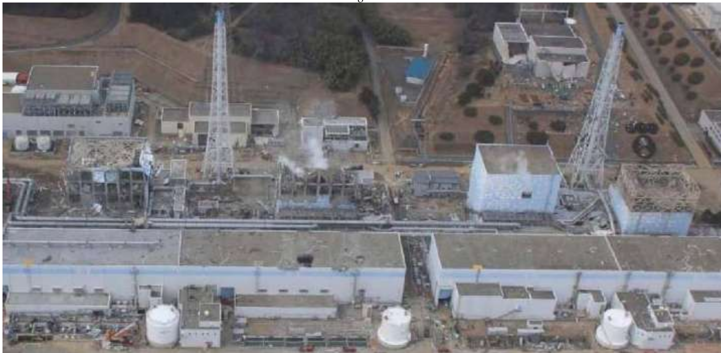
Photo of Fukushima Daiichi reactors 1-4 after the hydrogen explosions.
